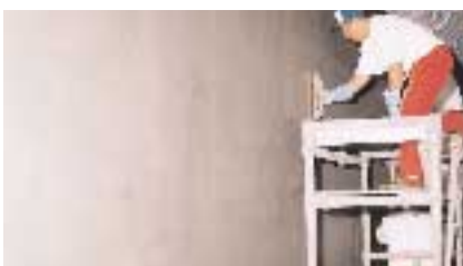
VANDEX CEMELAST as internal waterproofing.
