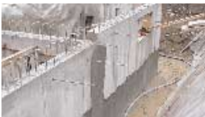
VANDEX CEMELAST as external waterproofing.
