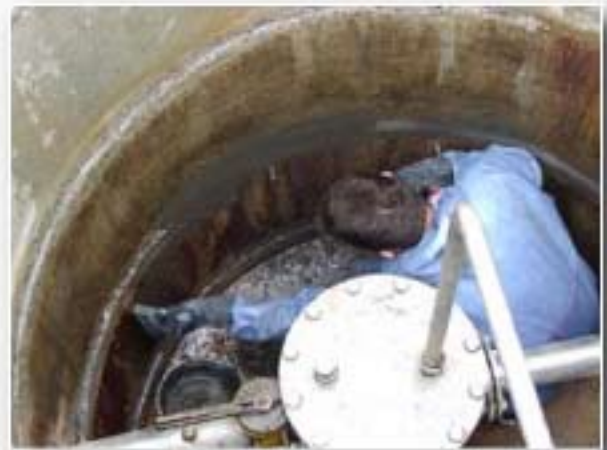
Sealing of leaking points
