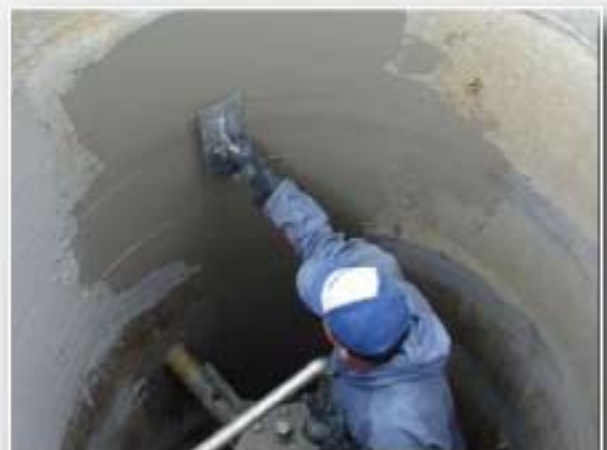
Waterproofing the surface
