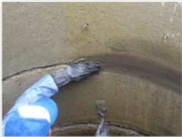
Sealing leaking joints
