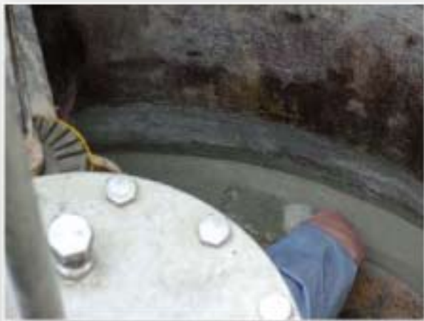
Applying a coved fillet at wall / floor junction
