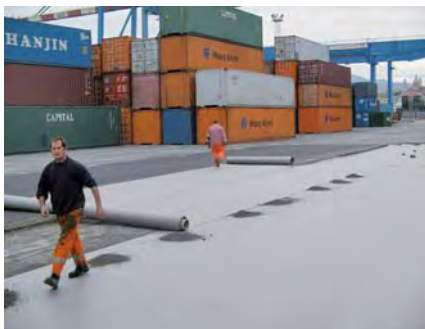
Posa Enkagrid® TRC
